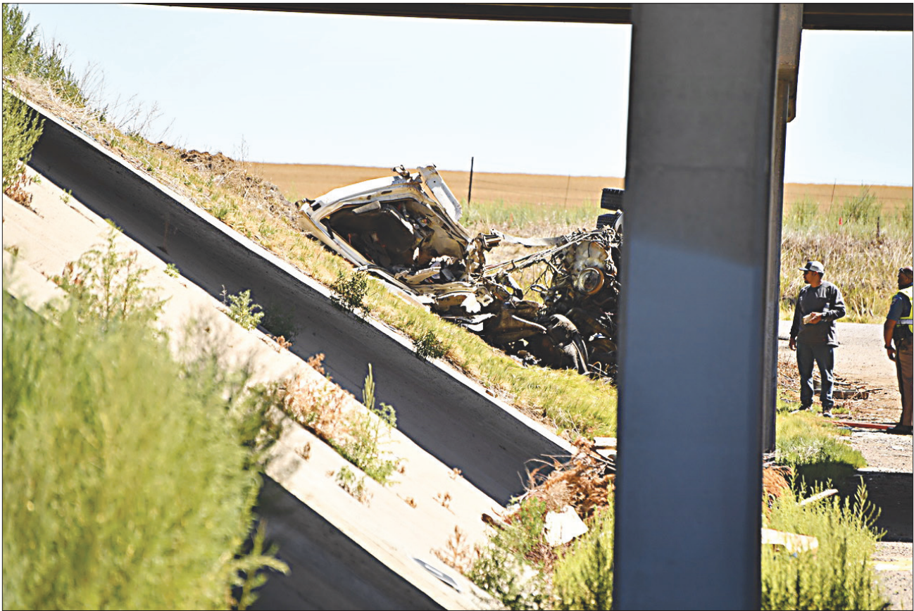
A 41-year-old Fort Morgan man miraculously evaded fatal injuries when the semi tractor-trailer rig he was driving crashed through a guardrail and came to rest on a bridge embankment on eastbound I-70 near mile marker 294 early afternoon Aug. 17. Above, the investigation of the wreckage continues after the driver was transported to a Denver hospital with serious injuries. SEE PAGE 4.
