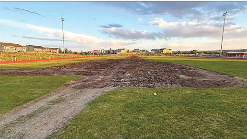
Among the summer projects on the Deer Trail School campus has been the replacement of much of the football field's grass. The new sod was originally planned to cover the area between the hashmarks in the middle of the field, but additional review revealed hard pan conditions throughout. The replacement occurred during the first week of June with hopes the new turf will be ready for the Eagles' first gridiron game Aug. 27 against La Veta.
