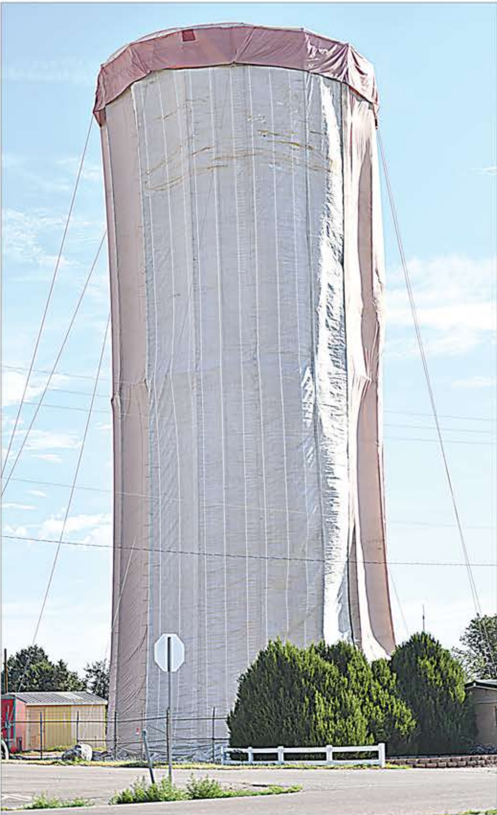
STEVEN VETTER/The I-70 Scout Last week saw the historic Strasburg elevated water tower go under the cover of a large tarp to prevent air contamination from the sandblasting portion of the tank improvement project. The inside of the tank is being re-coated and the exterior is receiving fresh coats of paint. Officials hope to have the tank back online by the first day of school on the Strasburg campus Aug. 6. The Strasburg Sanitation & Water District continues to urge customers to limit their outdoor irrigation until the project is completed and tank filled to capacity.
