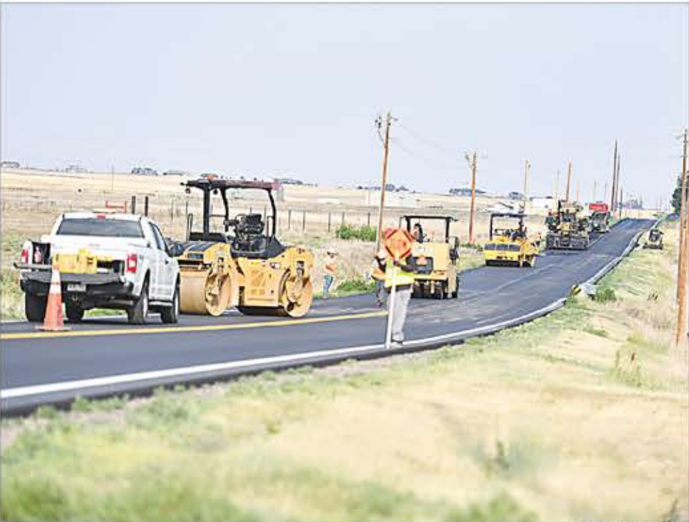
Asphalt improvements along 144th Avenue between Highway 79 and the 152nd Avenue curve about 10 miles north of Bennett are expected to be completed by the end of this week and similar work, starting with milling operations, was slated to occur on Piggott Road starting July 6. A third east Adams County paving operation along Strasburg Road from Colfax Avenue north to 48th Avenue will run concurrently. For more information, call (303)818.9854 or e-mail PublicinfoCO@gmail.com .
