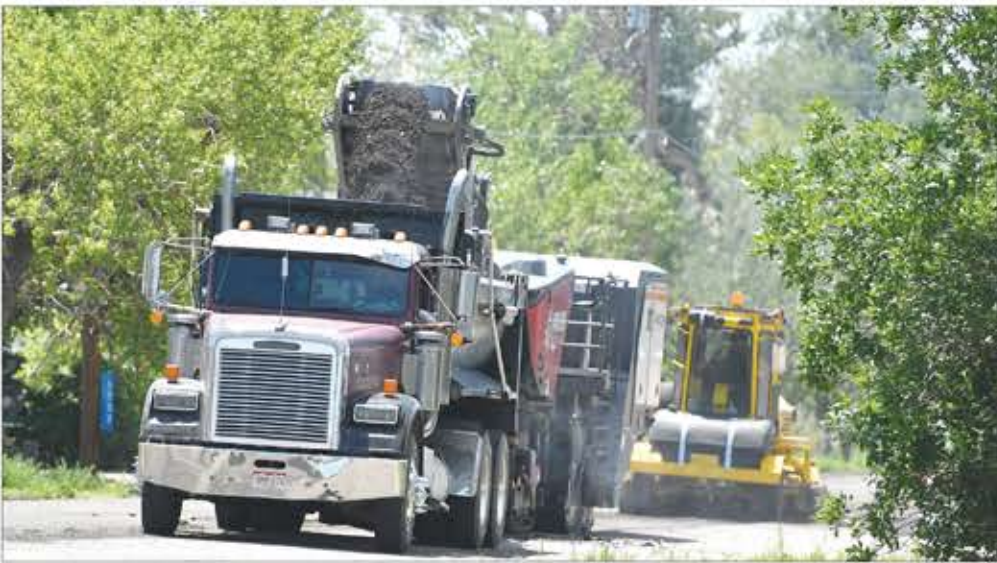
The milling portion of asphalt replacement along Strasburg Road between Colfax and 48th avenues began July 9. Work on the third of three east Adams County pavement replacement projects is expected to continue through at least this week and likely into next. The Strasburg Road project is concurrent with operations along Piggot Road and the Wolf Creek Run East subdivision on the west edge of town. Similar work has been done on 144th Avenue (Bromley Lane) between Highway 79 north of Bennett and the 152nd Avenue curve with Imboden Road north of Watkins.
