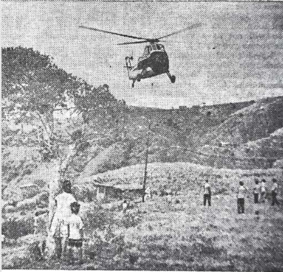
LIGHT WORK . . . Isolated Puerto Rican home gets electricity because a helicopter is used to lower a power line pole into a hole. Difficult terrain makes construction problems calling for the use of a helicopter.
