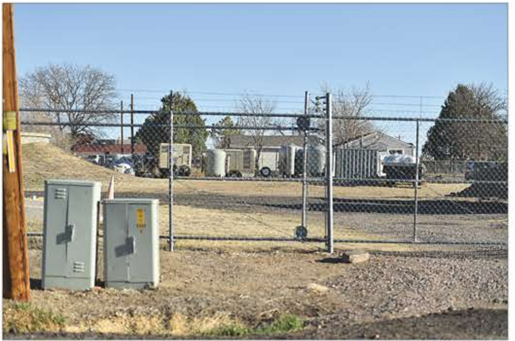
Some preliminary staging has occurred for the upcoming Strasburg water tower refurbishment project at the Strasburg Sanitation & Water District office yard next to the high school.
