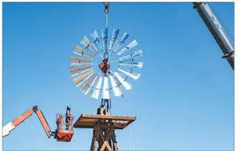
From left photo, workers attach the new Aermotor windmill to a crane for installation at the Arapahoe County Fairgrounds April 24; a crane lifts the new machine; and the windmill is lowered into place.
