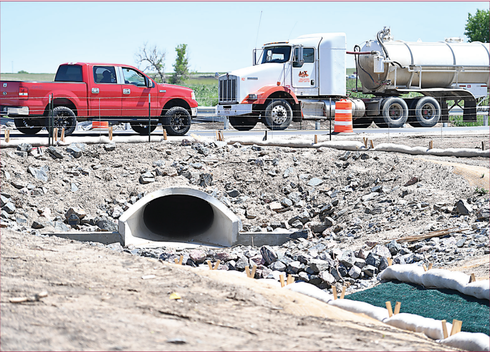
STEVEN VETTER/The I-70 Scout While drainage improvements have not been entirely completed at the interchange of Highway 36 (Colfax Avenue) and Kiowa-Bennett Road, intermittent traffic backups on both roadways came to an end in late May. The project includes installation of a new concrete culvert and widened drainage channels along the northbound side of Kiowa-Bennett Road and the eastbound side of Highway 36.
