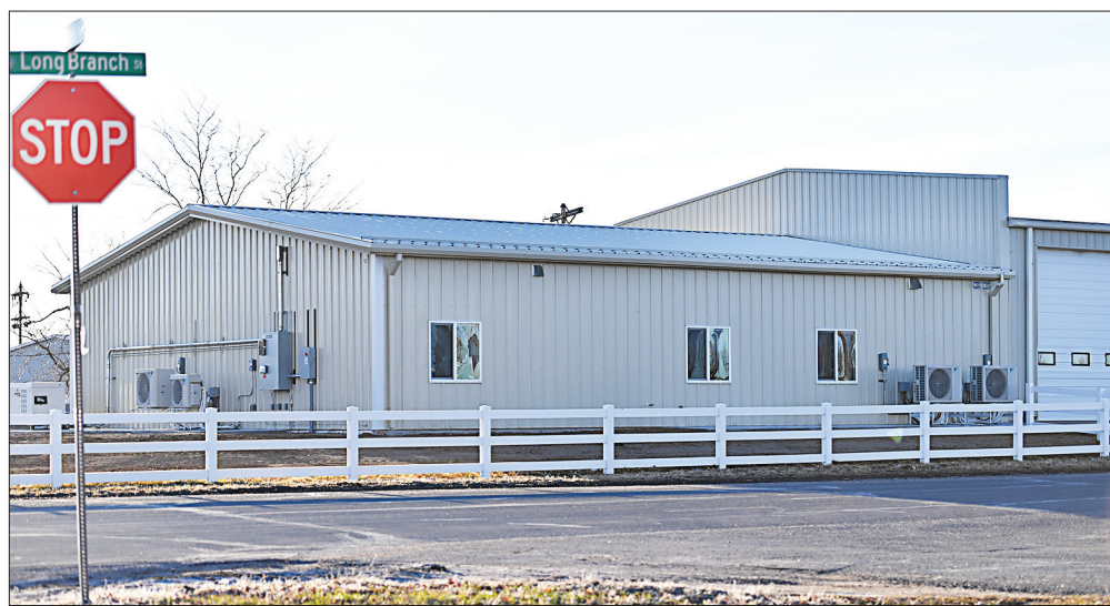
A grand opening of the new crew quarters, above, at the Strasburg Firehouse is tentatively set for the second weekend in May.
