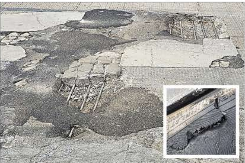
PHOTOS BY EMILY RICHARDSON/For The Scout Exposed rebar on eastbound/westbound I-70 about one mile east of the Peoria Road interchange punctured the tire of a Deer Trail woman last week.
